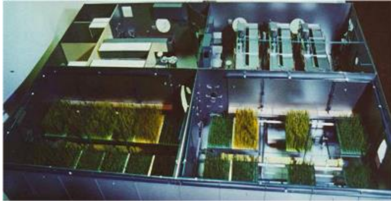
Figure 25 Scale model of Bios 3, Phytotrons are in front, crew quarters are in the upper left (Institute of Biophysics, 2019)
